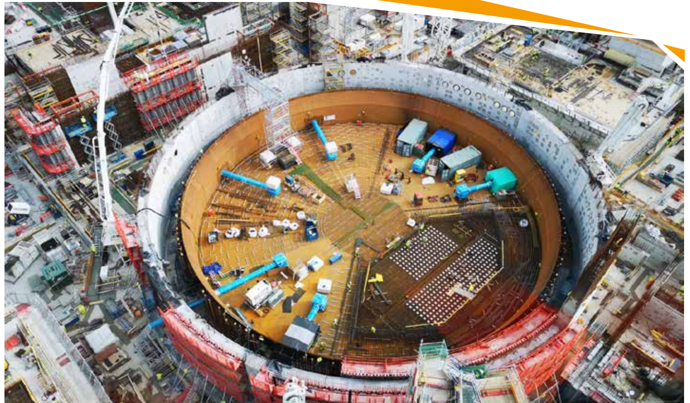
Unit 1 with liner cup and sump suction lines installed.
